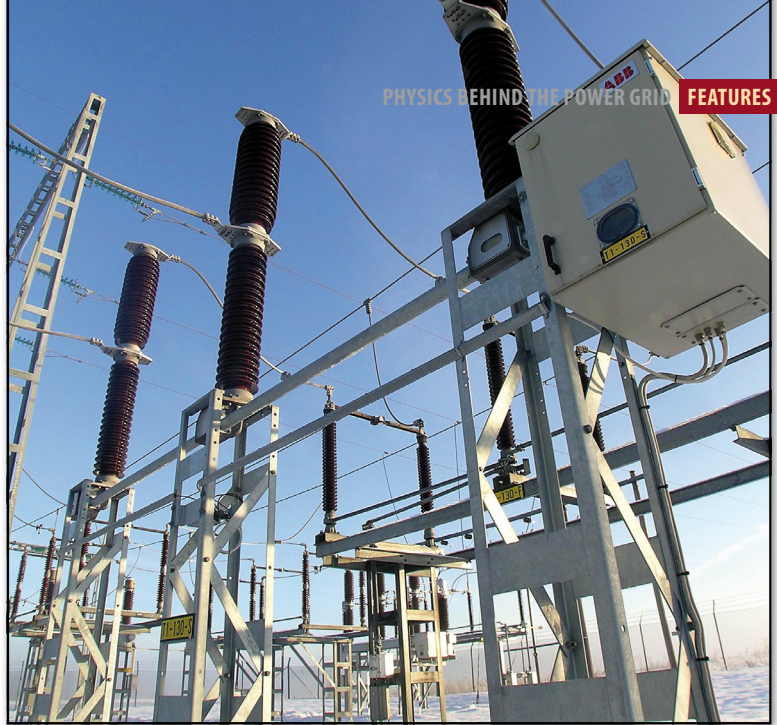
▲ FIG. 6. Three-phase high-voltage live tank circuit breaker. (Source: ABB)
