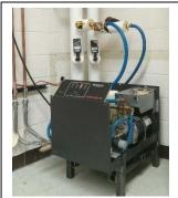
Figure 17: A Coherent LaserPure 20 chiller supplies chilled water to the Cryomech LHeP22. It is a closed-loop circulator chiller with a water pump and heat exchanger. The physics building supplied chilled water cools the heat exchanger.
