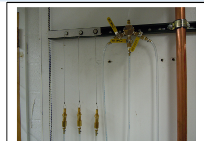
Figure 25: Lab dewar blow-off manifold
